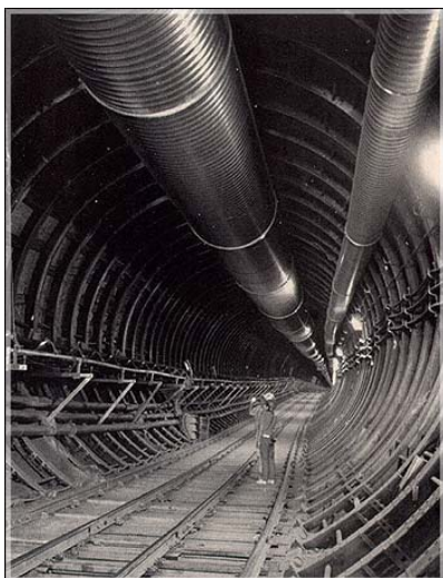
Yucca Mountain Tunnel
